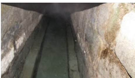
Figure 10: Figure 10. Hot water entering conduit 2 from the north.
