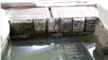
Figure 14: Hole in the wall from the castellum aquae into pool A.
