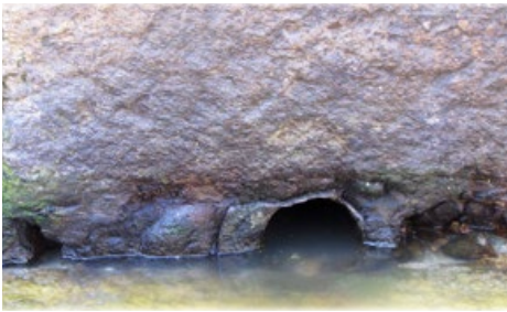
Figure 20: Lead fistula from pool A to cloaca 2.
