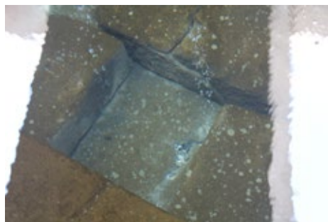
Figure 12: Thermo-mineral water coming out of the spring at the bottom of pool B.
