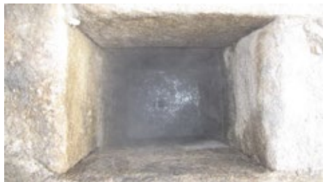
Figure 7: Inside of the Spring-well.
