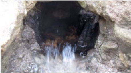
Figure 13: Wooden conduit that conveys the water into the castellum aquae.
