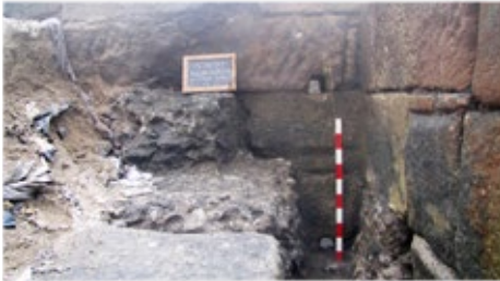
Figure 3: Opus caementicium substratum visible in the castellum aquae.
