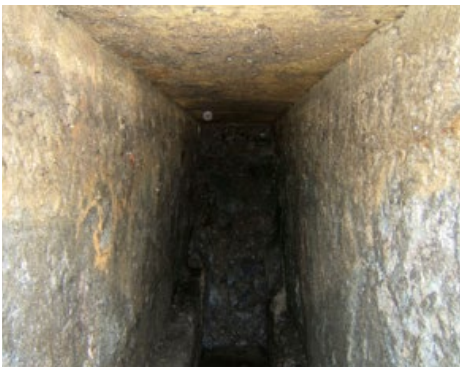
Figure 22: Opus signinum lining. Southern end of cloaca 1.
