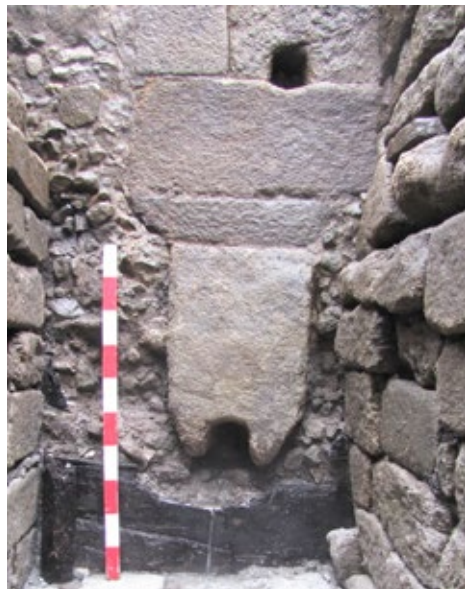
Figure 5: Opus caementicium substratum and wooden formwork visible under the masonry of cloaca 3.
